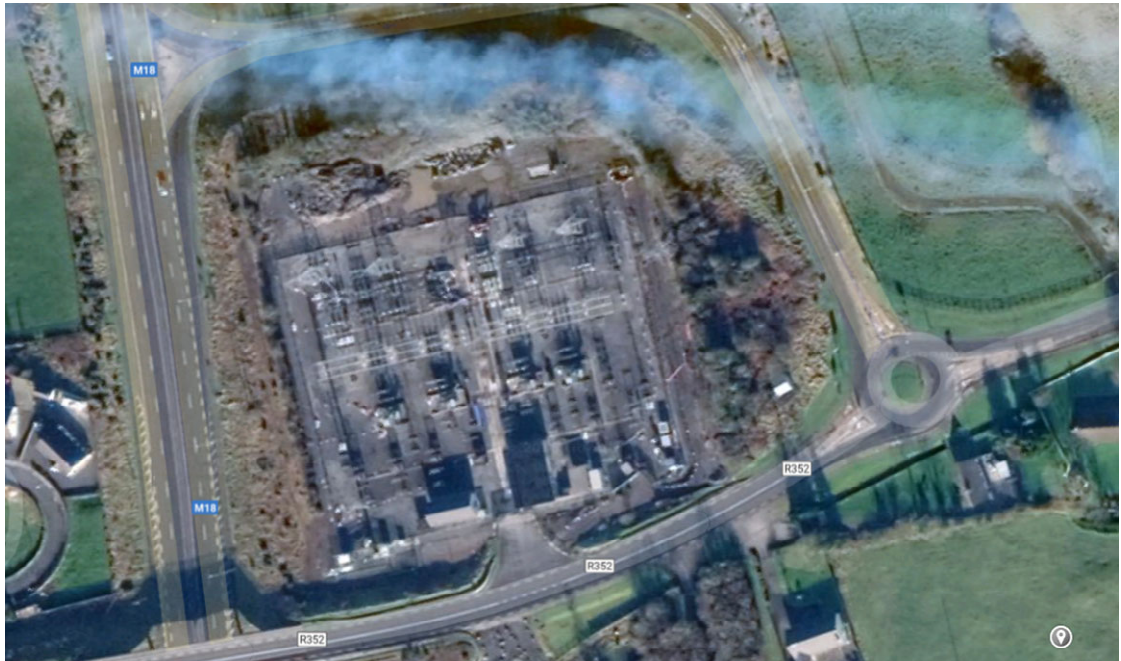
Figure 2-2. Ennis Grid Substation – Existing Physical Arrangement
